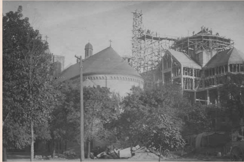
Remarkably, St. Joseph Chapel was completed in under four years.
